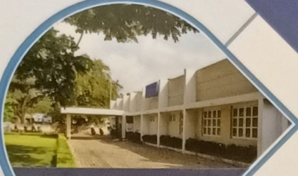
Hard Rock Regional Centre, Belagavi
