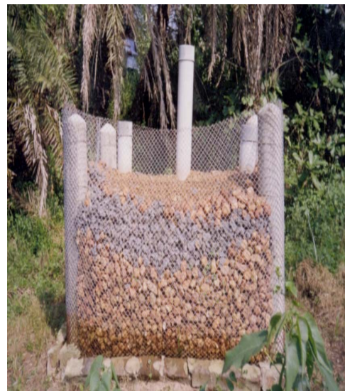
Fig.1:A Coastal Area (Krishna Delta) Fig. 2 Recharge well at Mopidevi
